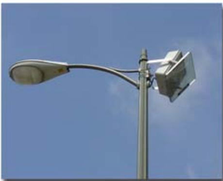
*Closed-circuit camera mounted on a light post.*
